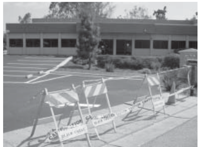
Preparation of the new Kelley Park Community Resource Center which opened in August.
